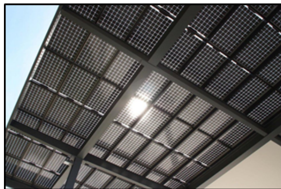
Bi-facial solar panels absorb reflected sunlight on the underside of solar panels increasing energy yields
