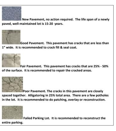
not continue to expand and contract. If cracks are ignored and not filled, you run the risk of your parking lot alligatoring. Alligatoring happens when cracks continue to spread throughout the entire lot- at which point you would need to have an overlay done or complete repave.
