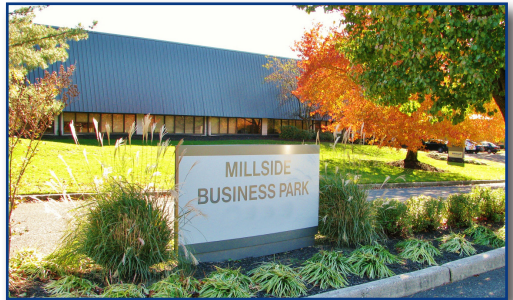
Millside Business Park 1835 Underwood Blvd. | Delran, NJ
