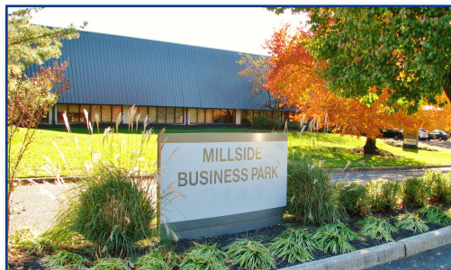
Millside Business Park 1835 Underwood Blvd. | Delran, NJ
