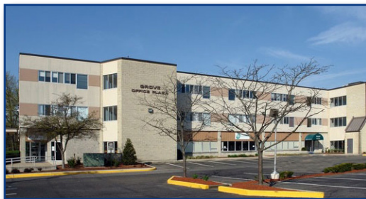
515 Grove Street | Haddon Heights, NJ
