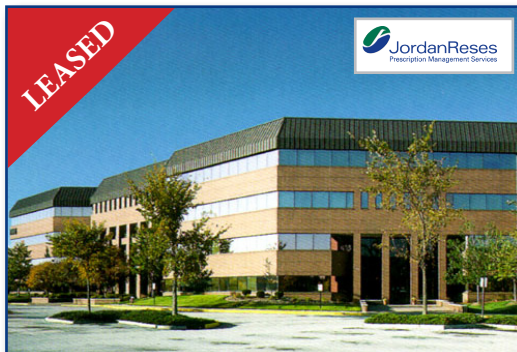
Five Greentree Centre | Marlton, NJ
