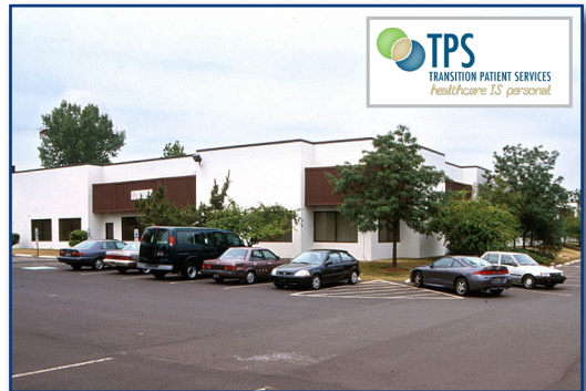
Metropolitan Business Center 2540 Metropolitan Drive | Trevoese, PA
