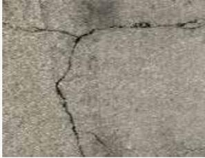
Good pavement. This pavement has cracks that are less than 1". It is recommended to crack fill & seal coat.
