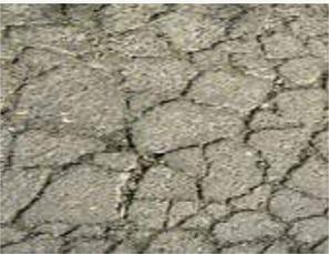
Poor pavement. The cracks in this pavement are closely spaced together. Alligatoring in 25% total area. There are a few potholes in the lot. It is recommended to do patching, overlay or reconstruction.
