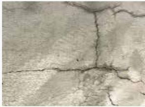
Fair pavement. This pavement has cracks that are 25% - 50% of the surface. It is recommended to repair the cracked areas.
