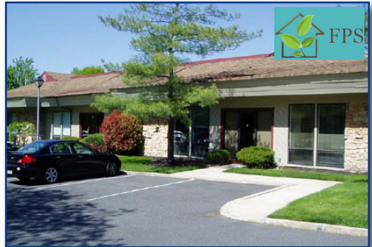
Greentree Commons 951 Route 73 North | Marlton, NJ
