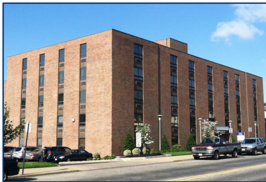
Station Office Building 900 Haddon Avenue | Collingswood, NJ
