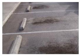
Protect against gasoline oil spills from automobiles that damage and soften the surface.
