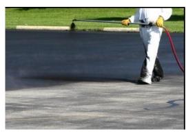
Properly applied, sealcoat can save an owner huge costs over the life of a hot mix asphalt pavement.
